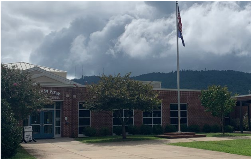
Mountain View Elementary School.
