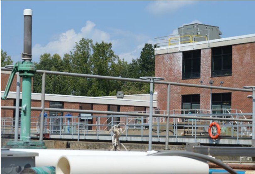
The South Rivanna Water Treatment Plant (RWSA).
